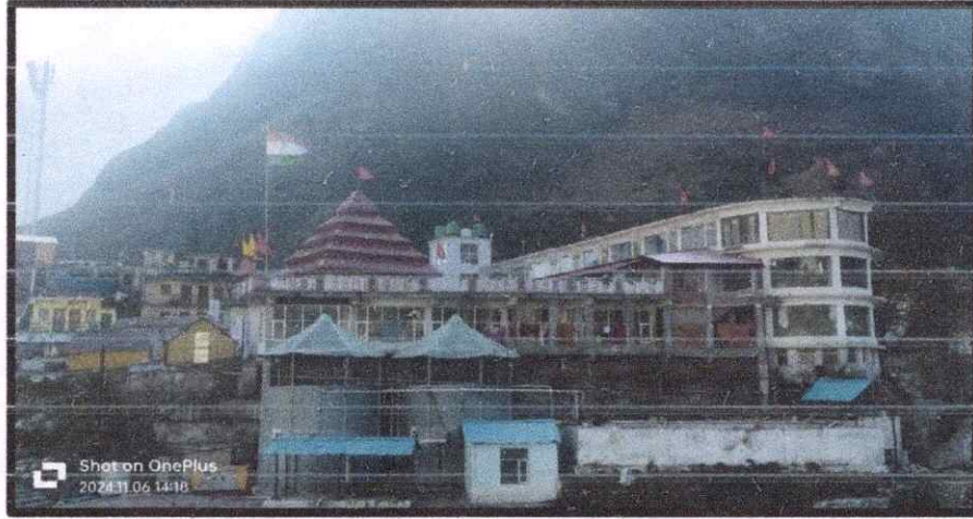
0.26 MLD STP near Bamani Gaon
