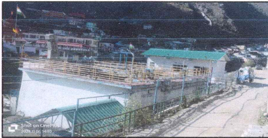
1.00 MLD STP near Suspension Bridge
