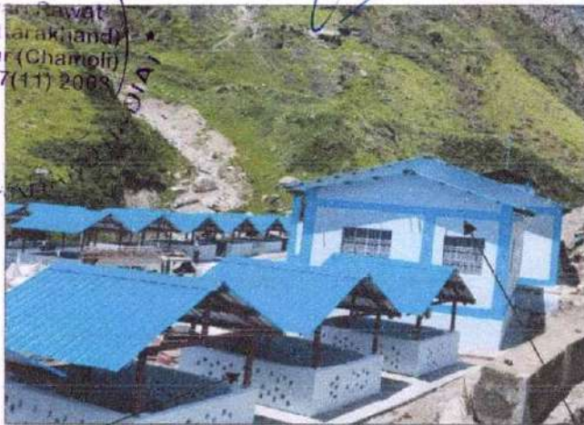
Nadep Pits (10 no.)
